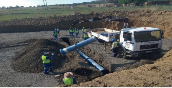
Installation of inlet pipes for New Clarifier Tayside, Dundee.
