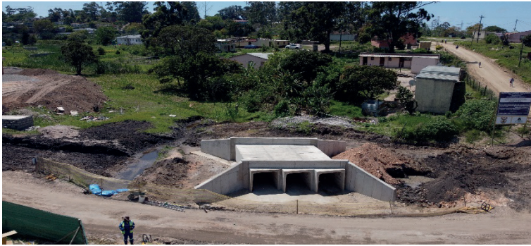
Construction of portal culverts at KwaSithole vehicular bridge & Concrete Road.
