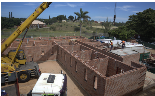
Placing of pre cast slabs
