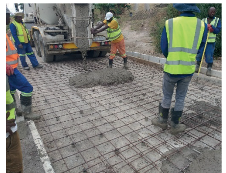
Construction of concrete access road at Kwa Sithole in Portshepston/ Ray Nkonyeni Municipality.
