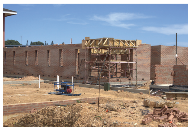
Brickwork at wall plate level
