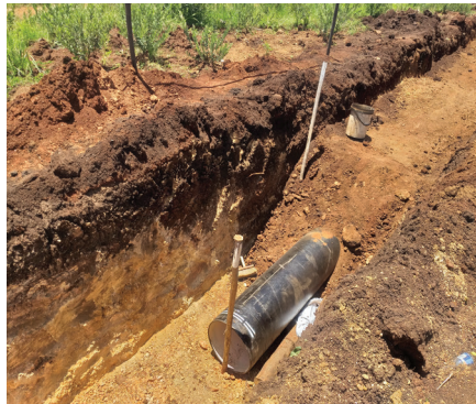
Laying of ductile pipe
